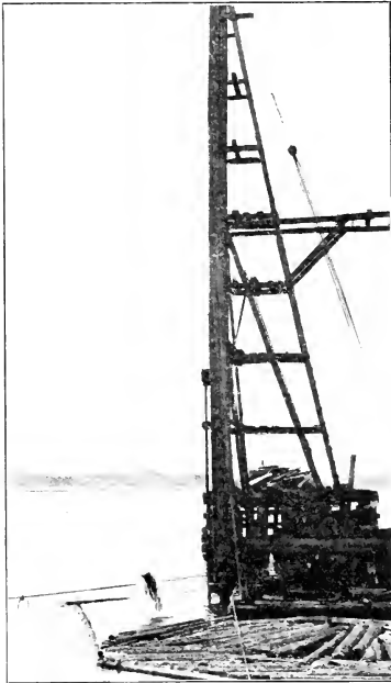
FIG. 17. CUTTING PILES FOR HARBOR PIERS.
